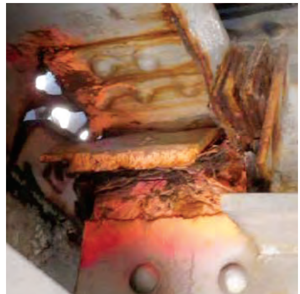
Deterioration at expansion joint support
