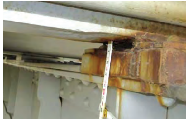
Typical deterioration at steel elements
