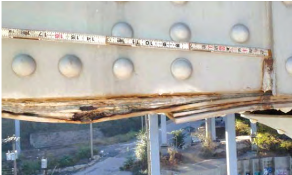
Extensive corrosion at the approach piers
